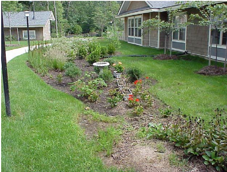
Bioretention Filter in multi-family residential setting
