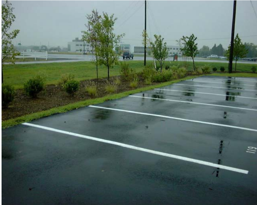
Bioretention Basins in office setting parking lot
