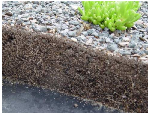
Figure 3 Photos of Vegetated Roof Cross-Sections (source: B. Hunt, NCSU)
